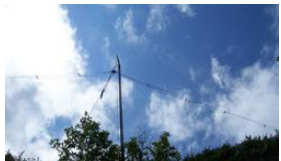
Figure 2: The center of the inverted V raised into position at the top of the Unistrut support.
