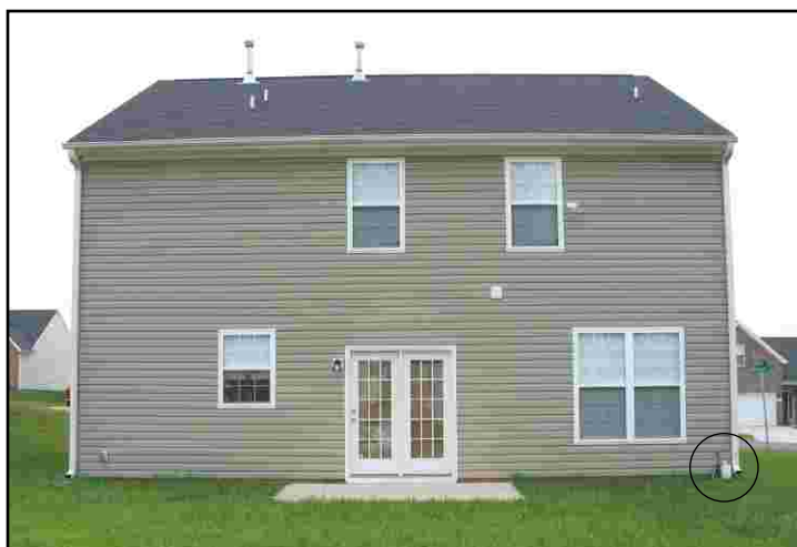
Gutter Set-up - The left photo shows the set-up of N8NQP's gutter antenna and the photo above is the back of his house with the gutter running the full length. The circle indicates the antenna coupler.
