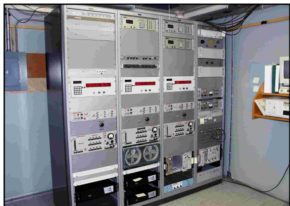
Above, the time code generation room at WWV. This is a shielded room that holds the three — primary, secondary and tertiary — time code generators and digital announcers used for the WWV stations. At the right, two of the three Continental transmitters used by WWV/B. Each transmitter outputs 38 kW of RF, and each feeds a separate antenna. Together, the two WWV/B antennas are fed in phase to form a directional antenna, concentrating the signal to the east/southeast.
