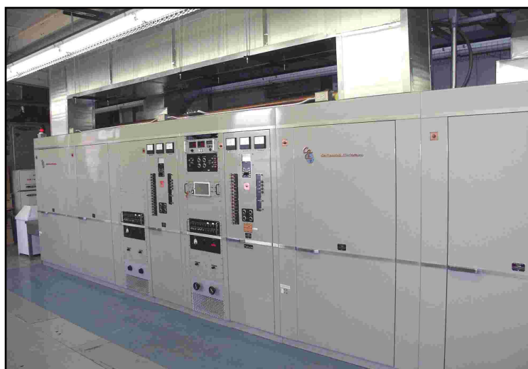
Above, the time code generation room at WWV. This is a shielded room that holds the three — primary, secondary and tertiary — time code generators and digital announcers used for the WWV stations. At the right, two of the three Continental transmitters used by WWV/B. Each transmitter outputs 38 kW of RF, and each feeds a separate antenna. Together, the two WWV/B antennas are fed in phase to form a directional antenna, concentrating the signal to the east/southeast.
