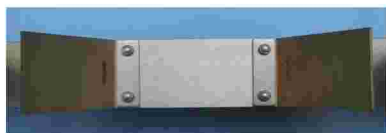
Photo 2a - Original braces (with rivets)
