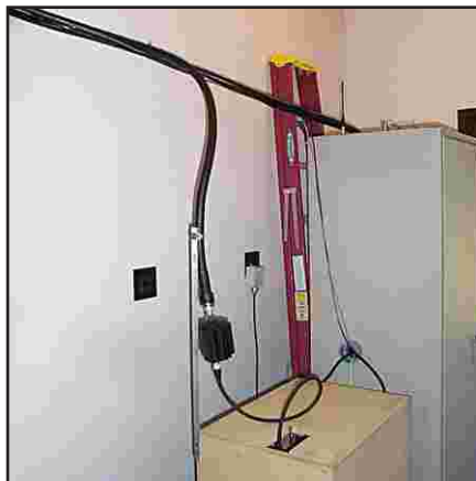
Feed lines attached to wall duplexers box. (Photo by N4DFA)
