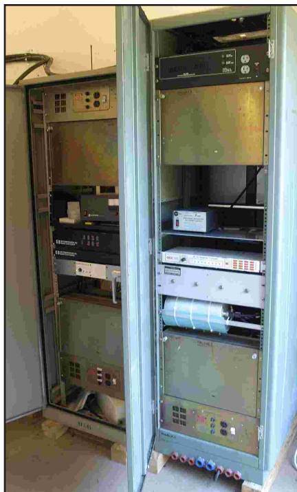
Two-meter repeaters on left and the new 440 machines on right. (Photo by N4GVK)
