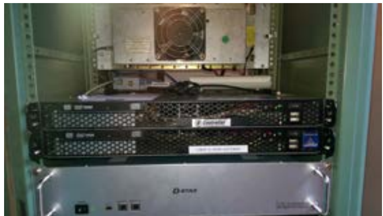
Removed 4ft long Ethernet jumpers and replaced with 1ft jumpers to clean up the install a bit.
