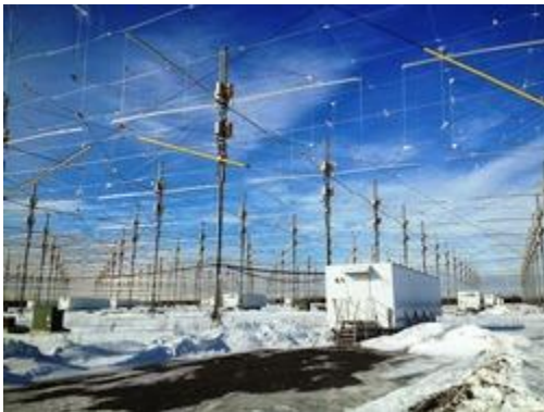
Part of the massive antenna field at the HAARP facility near Gakona, Alaska. The row of white structures contains individual transmitters.
